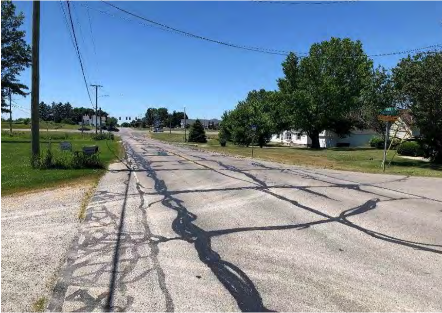
Photo 53. Facing west toward SR 3, along southside of Drake Rd.
