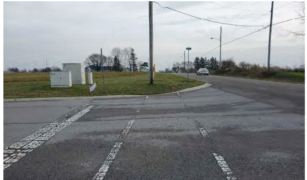
Image 4: Intersection of Drake Rd and Glory Ave facing east.
