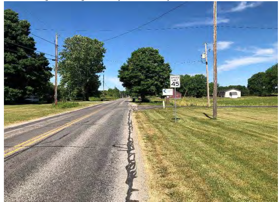
Photo 4. Facing west along northside of Drake Rd from western terminus of the investigated area.
