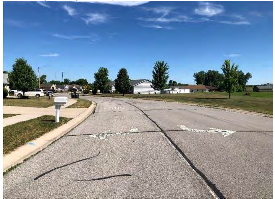
Photo 8. Facing north along Glory Avenue from northside of Drake Rd.
