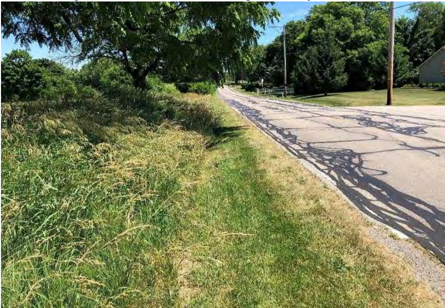
Photo 58. Facing east toward eastern terminus of the investigated area, along northside of Drake Rd.
