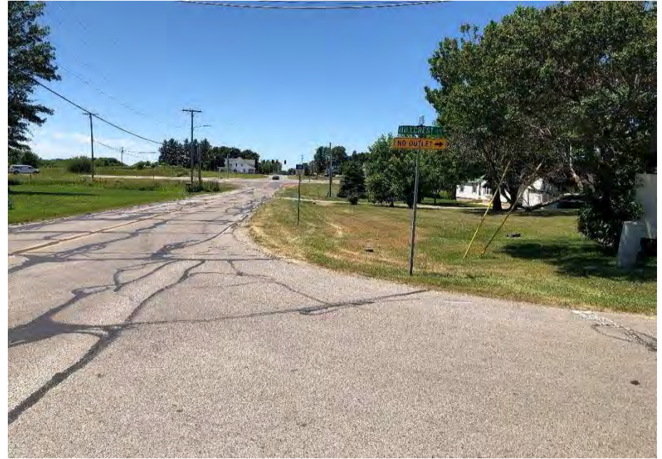
Photo 55. Facing west toward SR 3, along northside of Drake Rd from Hillcrest Dr.
