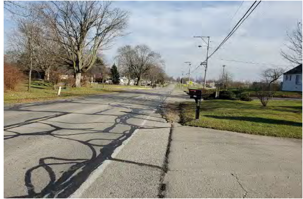
Image 10: The intersection of Drake Rd and Briarwood Dr, facing east.
