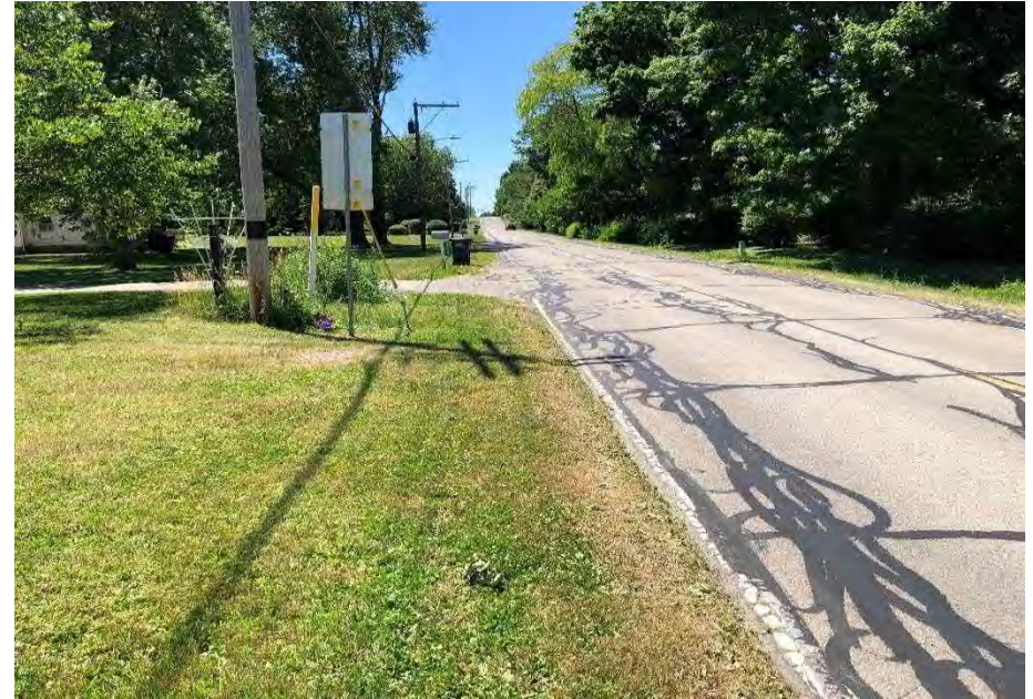
Photo 71. Facing west along southside of Drake Rd.
