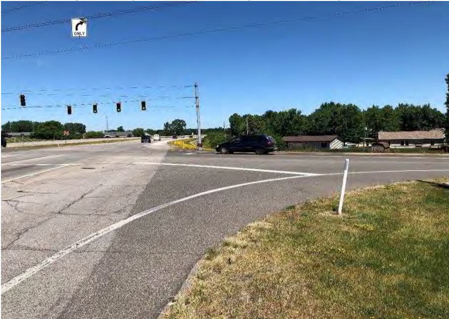
Photo 42. Facing north toward Drake Rd from southeast corner of the intersection of Drake Rd and SR 3.
