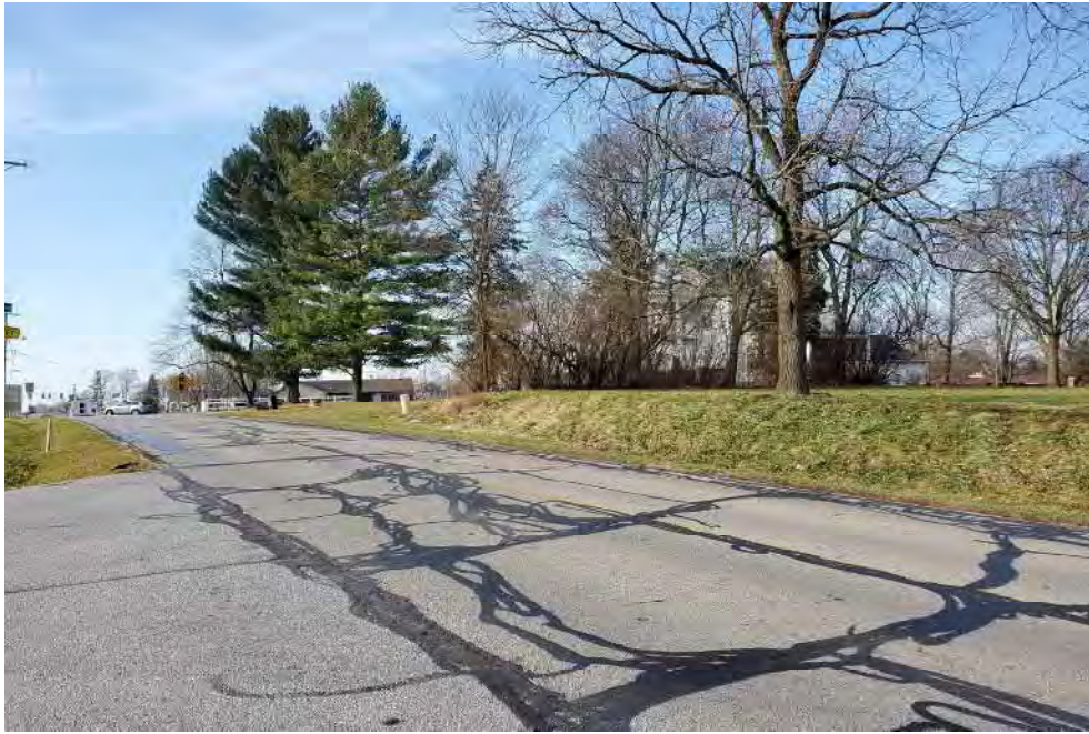
Image 9: The intersection of Drake Rd and Bison Blvd, facing west.
