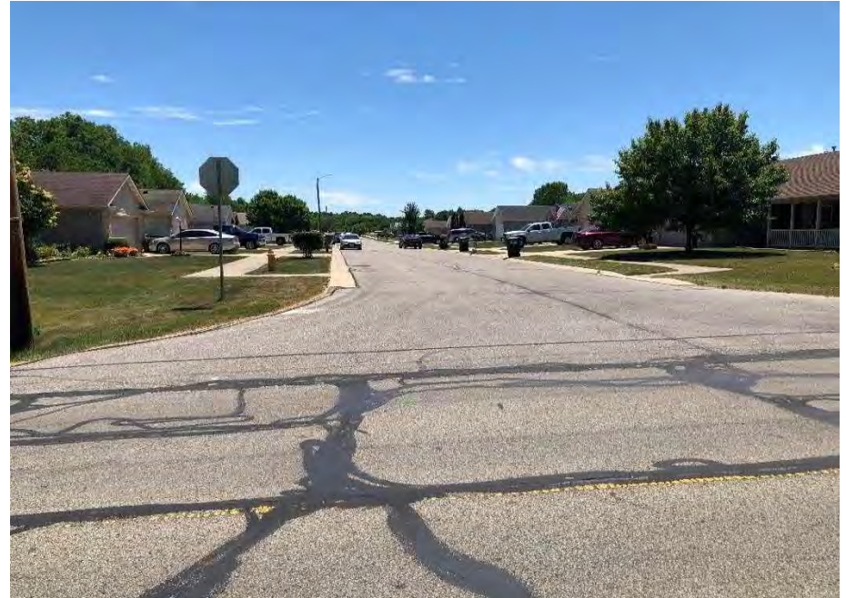
Photo 59. Facing south along Bison Boulevard from northside of Drake Rd.
