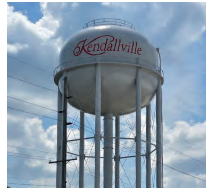
Part of the system that gives Kendallville room to grow – one of the City's three elevated water towers.
