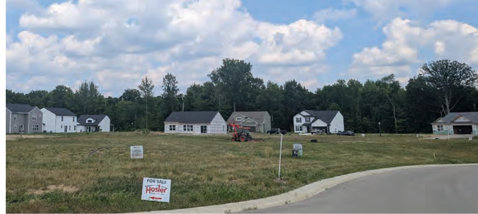
Noble Creek Subdivision on the City’s southeast side will ultimately include 72 lots, with construction underway on the 33 lots that make up Section 1.
