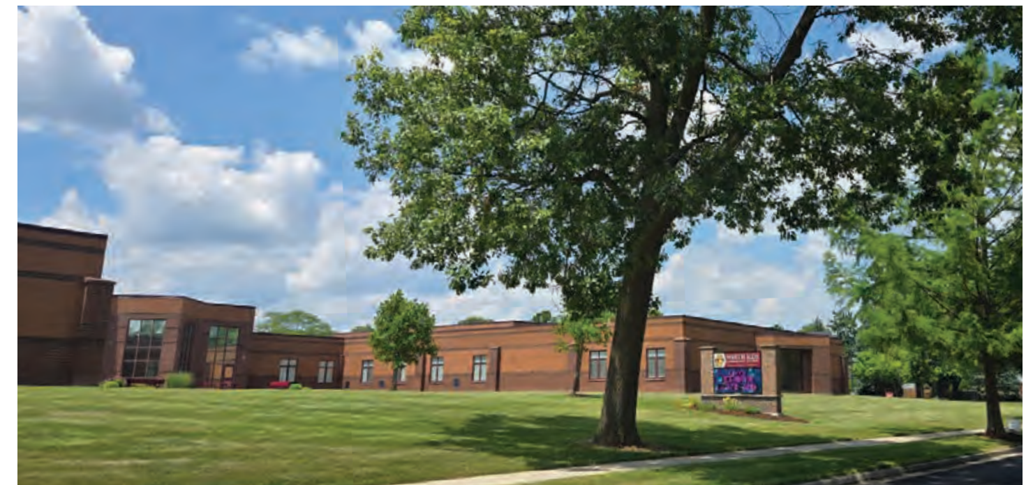
North Side Elementary School is a good example of a transitional land use. It's presently zoned R-1 (Single Family).
