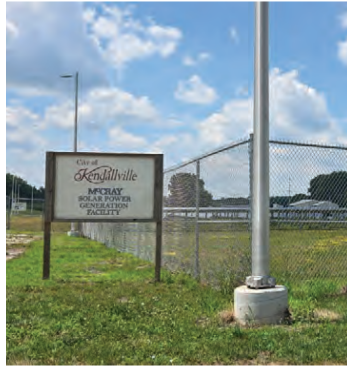
Above: The City constructed a small solar field on the former site of McCray Refrigeration and named the site accordingly. Below: Google Earth illustrates the size of McCray Solar Power Generation Facility and its proximity to the City's Wastewater Treatment Plant.
